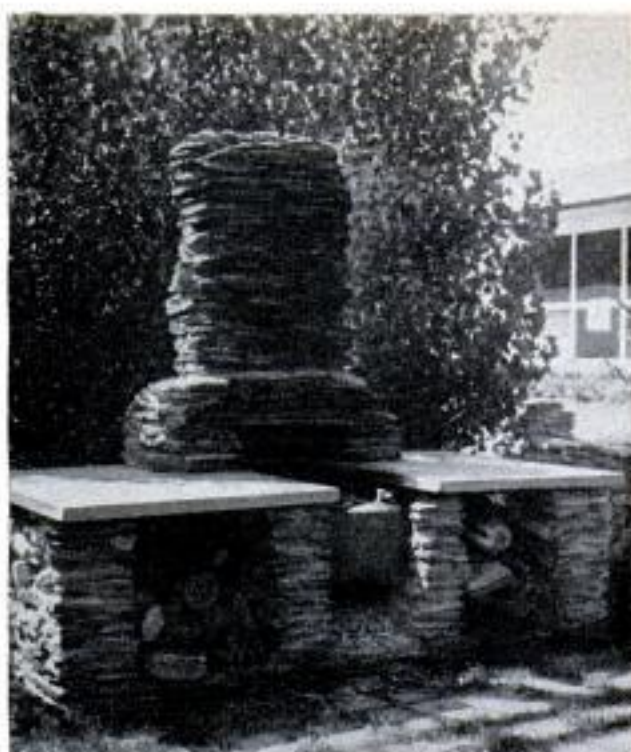
Sandstone slabs top fuel-box tables of shale fireplace
